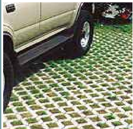
Pervious surface is ideal for overflow parking - Center for Watershed Protection
