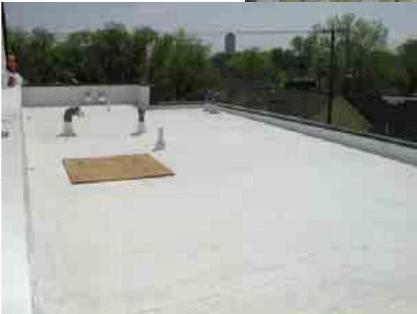
White roof surface reflects heat in summer to reduce cooling demand.
