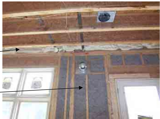
Caulked and sealed building envelope - windows and wall studs
